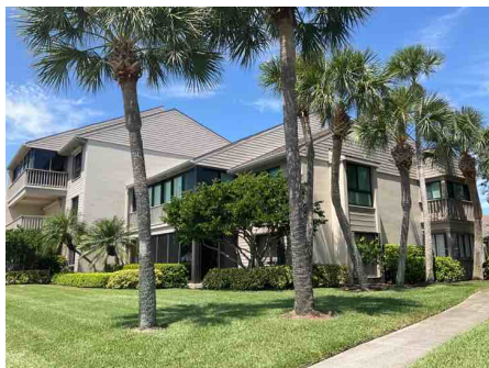
Elevation and unprotected glazed openings
