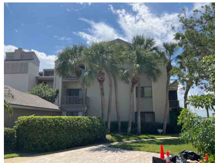
Elevation and unprotected glazed openings
