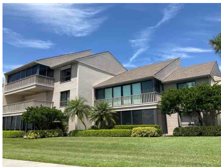
Elevation and unprotected glazed openings
